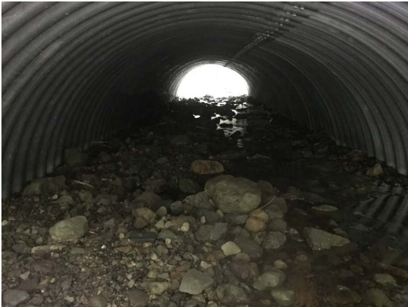
Looking through culvert
